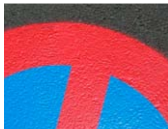
Closeup shot - showing adhesive conforming to asphalt.
